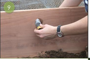
Use the additional hardware to build a connector between your PVC pipes and your garden hose. The connector should be high enough to allow the PVC garden hose adapter to run through the hole you've just drilled.
