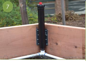
Place your pop-up sprinklers into the PVC at each corner of the garden. The top of the sprinkler should be at least six inches above the top of the garden walls.
